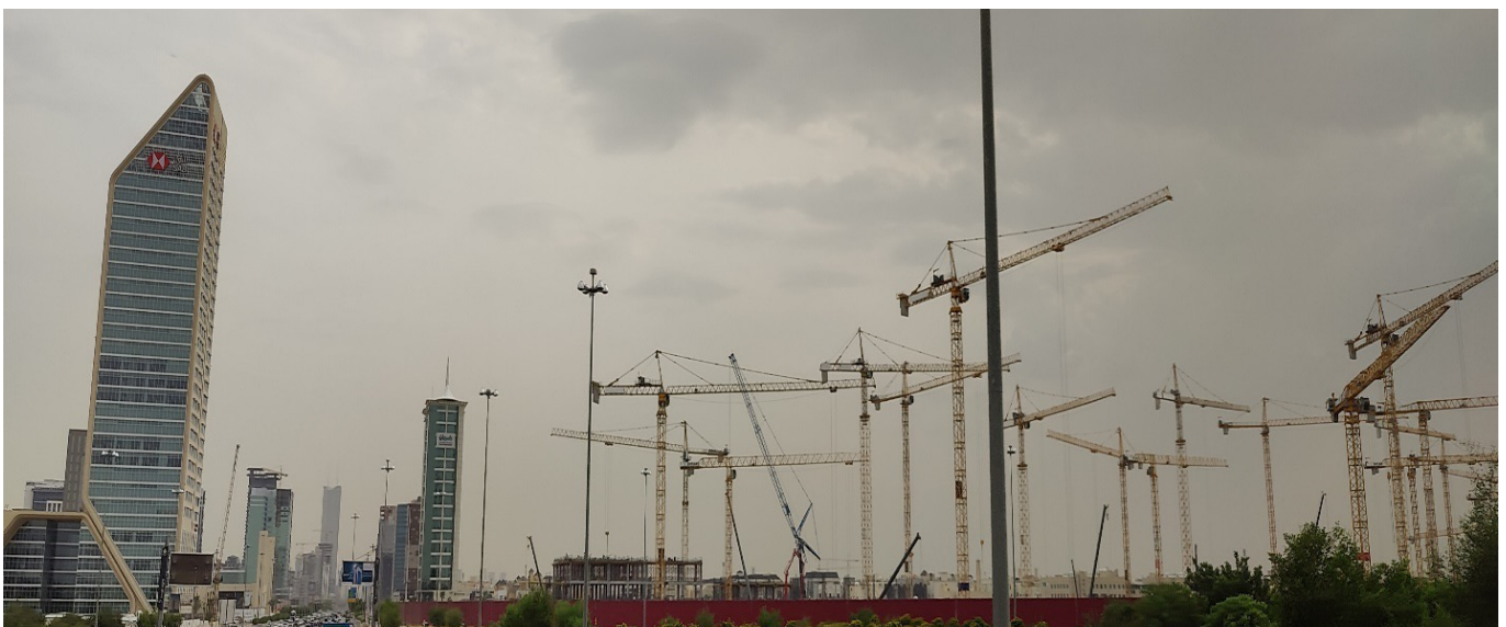
Riyadh under construction.
